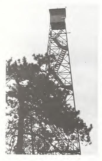
Figure 200. Grandview lookout, an Aermotor MC-39, is 80 feet tall and was built in 1936.
